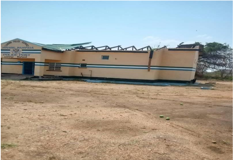
Figure 4 Renovation of a police post
